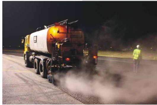
The Repave process also treated the cracks in the underlying runway surface which were still present after the initial planing operation negating the need for a separate repair prior to surfacing. The runway was grooved after 48 hours and in order to facilitate this, other works were programmed on adjacent taxiways on alternate nights.
