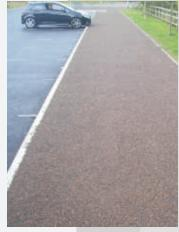
The introduction of chopped glass fibres in the process gives the surface the extra tensile strength and flexibility that is needed to cope with the pressures and stresses exerted on the surfaces by cyclists and pedestrians.
