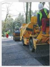
Fibredec's bespoke smaller plant was ideally suited to laying the product on the relatively narrow pathway through the woodland track and particularly so when faced with the narrow bridge spanning the brook.
