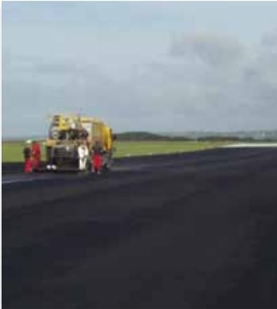
Bitutex is a low cost, high quality, cationic slurry surfacing veneer carpet of coated fine aggregate. It is ideal for housing estate roads and car parks where it provides a clean, dense, sealed surface as an alternative to surface dressing. It is also suitable for airfield use.
