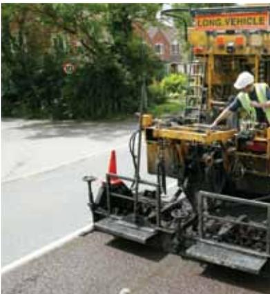
Based on well-tried German technology and extensive UK contracting experience, Ralumac 1000 fills ruts, restores profile and treats a deteriorating road surface.
