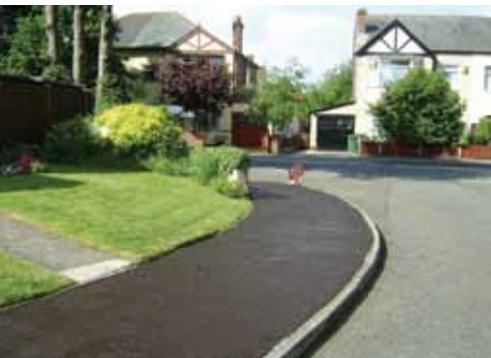
Colas supplies a range of slurry surfacing and microsurfacing treatments, designed to improve the appearance of any footway and reduce the number of trips and alleviate the ingress of water, thereby preventing further damage.
